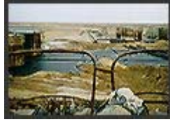
Land spill at tank farm
